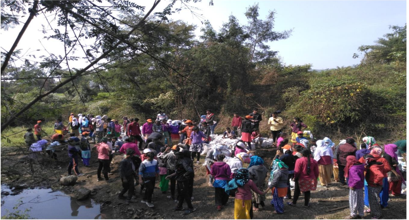
Construction of Vanrai Dam at Kurwandi village Date: 17/12/2017
